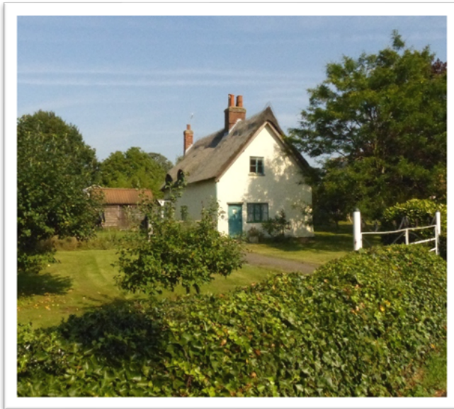
One of several attractive cottages in the village, an intrinsic element of Ickleford's identity
